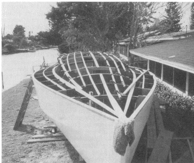
most of the hardware and cleats himself. Construction is marine plywood over full-length fir stringers, covered with Fibreglass and epoxy. Launching was in November 1989, he reports, when "with the help of twenty friends and twenty pounds of lard we skidded her over the seawall into the canal."
