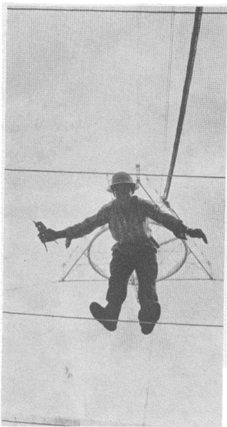
Worker attaches reflector mesh to cables.
