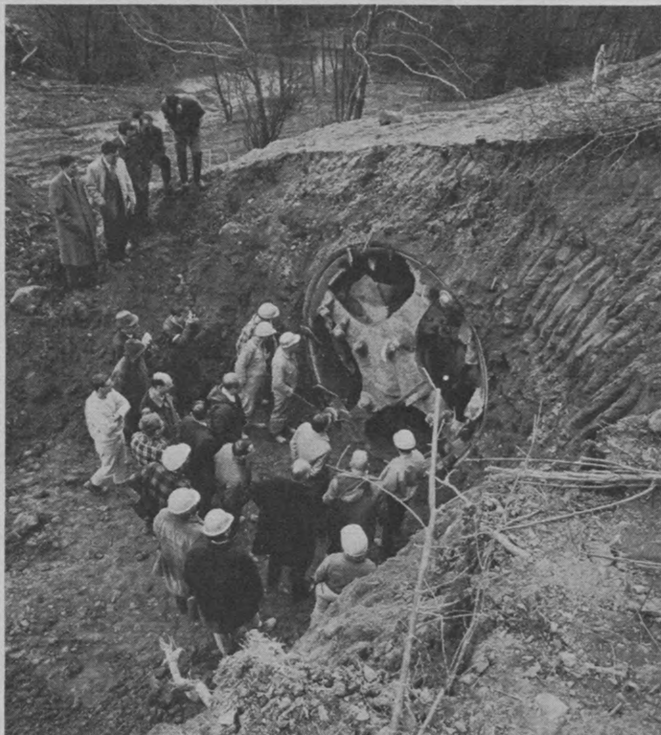
Physicists, builders, and business managers watch as the tunneling machinery emerges from under Upper Alumni Field completing the first stage of synchrotron construction.
