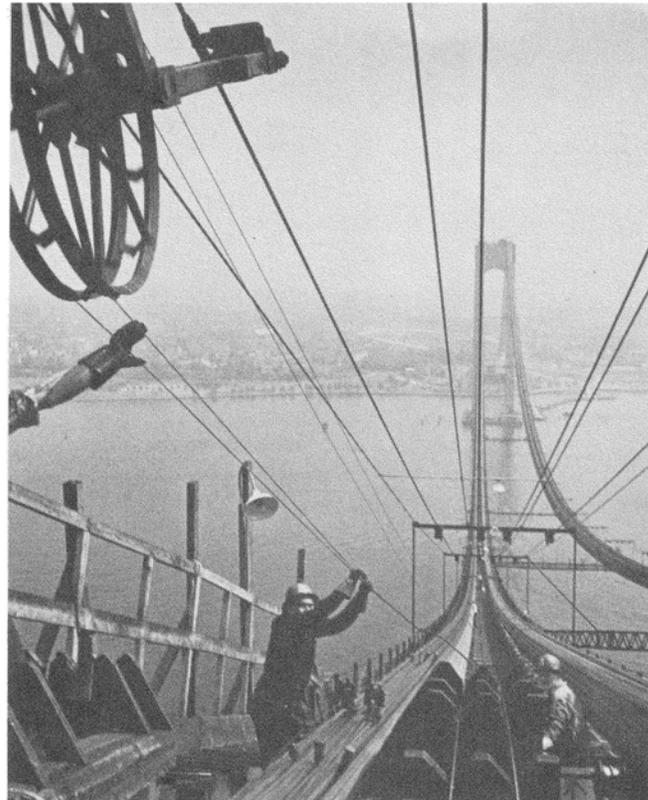
Towers (left) and cable spinning on Narrows Bridge, 1963.
