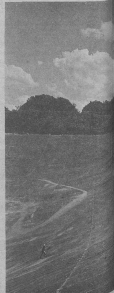
VERY BIG DISH — The fixed reflector very big indeed: it is 1,000 feet in diameter. The worker trudging up the side of the dish distribute his weight over the surface of the dish.
