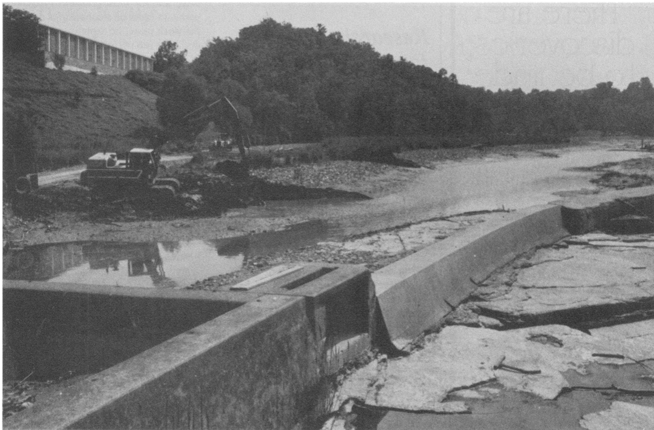
A backhoe moves silt in a drained Beebe Lake. Silt will be used to build up eroded shore and the island at the far end.
